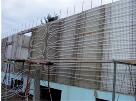
FIGURE 4. The external partition with an active thermal insulation (photo by BT&SONS Kft, 15 April 2017)
