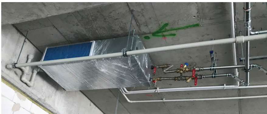
FIGURE 6. The heat pump (WLHP) connected to the water installation by the pipe system with the control valve, the sieve filter and shut off valves (author: Dorota Leciej-Pirczewska)
