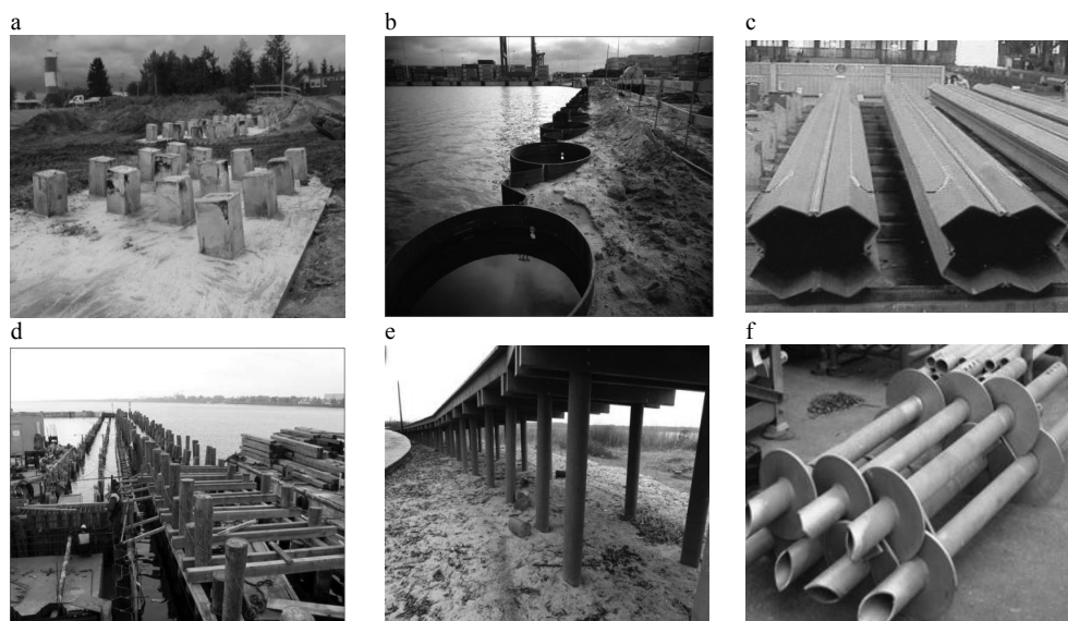
FIGURE 2. Types of piles: a – prefabricated reinforced concrete piles (photo by K. Gwizdała); b – pipe piles (photo by K. Gwizdała); c – steel profile piles (©Thyssen Krupp); d – wooden piles (photo by K. Gwizdała); e – plastic piles (©Akerpol.pl); f – disc screw pile (©sw.birmiss.com)
