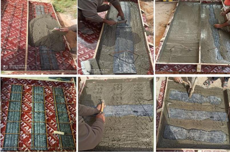
FIGURE 4. Reinforcement and DTS fixing processes and concrete casting for the RCOWS and RCTWS models
