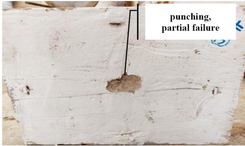
FIGURE 15. Failure pattern of 18 cm slabs with two layers of geogrid at 3 cm after impact loading Source: own work.
