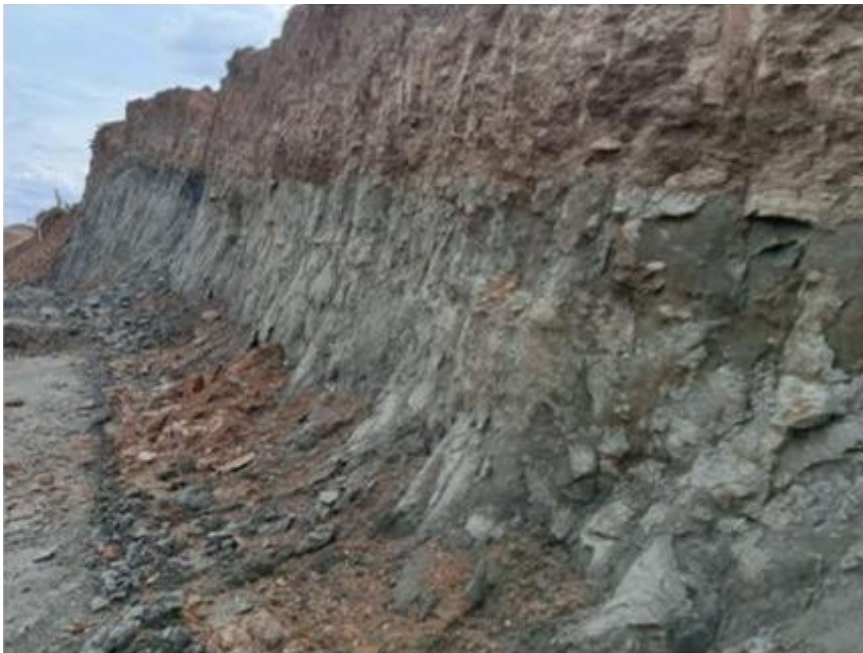
FIGURE 1. Clay shale slope in toll road project in Indonesia
