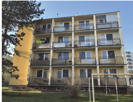
FIGURE 1. View of a point-access panel building
